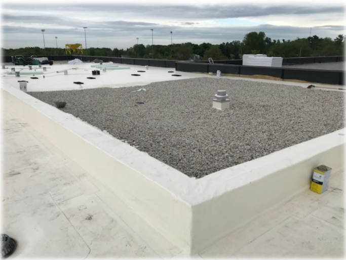
New Middle School Roof
